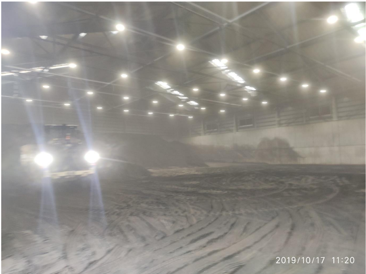
Hibikinada: Covered coal yard
