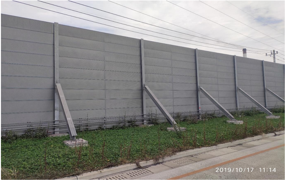
Hibikinada: Modular perimeter wall
